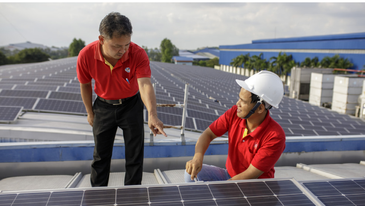
Solar Plant Sao Mai Corporation Vietnam © GIZ / Thomas Imo
